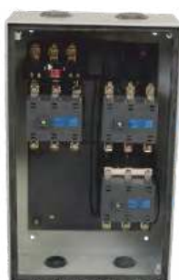
Interior View of ML SASD
