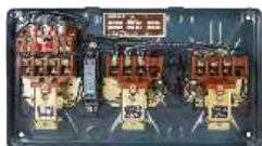
Interior View of MK2 FASD
