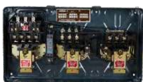
Interior View of MK1 FASD
